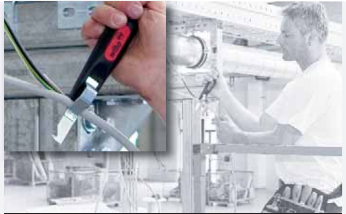
Cutting back of cables.
