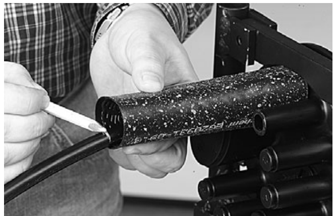
4.2.3 Remove the packing bag out of the seal, push the seal upwards to base and mark the cable.
