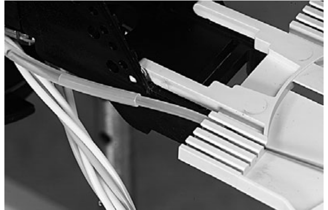
5.3.5 Install the FOPT in the tray. The FOPT CT should overlap both tubes around 30 mm.
