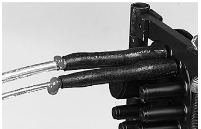
4.2.9 Install the seal.
