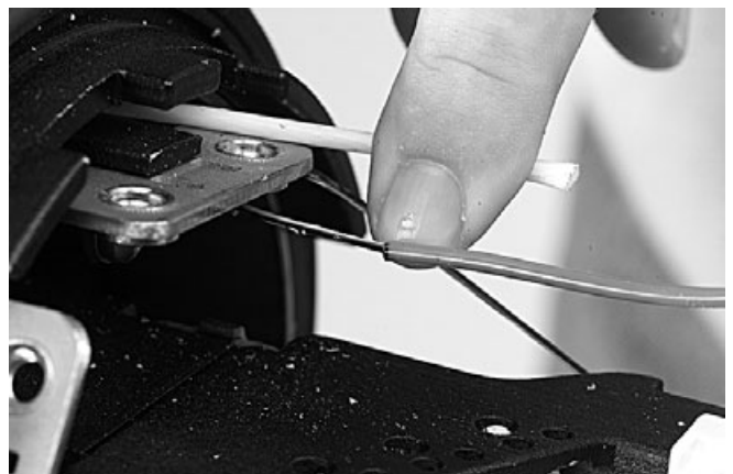
3.2.9 Strip the loose tubes that are already prepared to be stripped.
