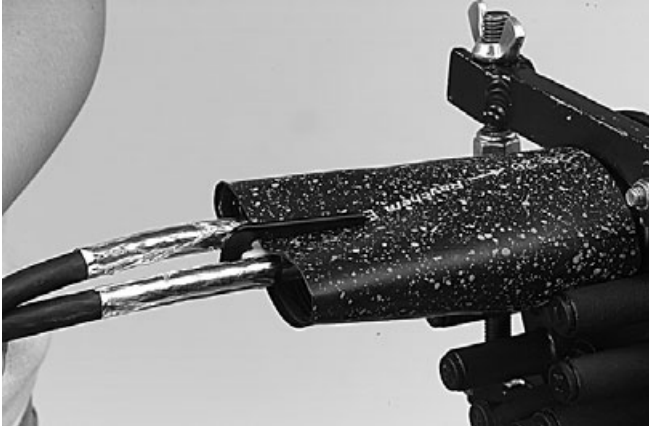
4.1.5 Push the seal against the base and place the clip.
