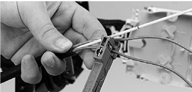
3.2.6 Already make a groove in the tubes at the mark. Prepare the loose tubes to strip afterwards inside the closure. Important: place the tubing over the cable before pushing the cable into the closure, check the arrow on the tubing, pointing towards the base.
