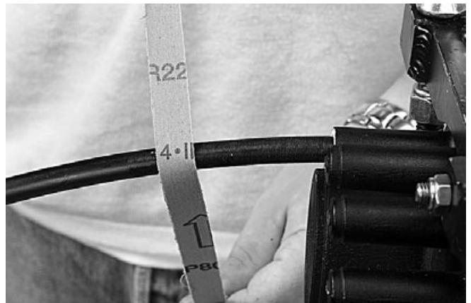
4.2.2 Abrade cable and round port.
