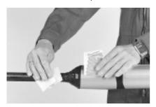
**10** Remove solvent impregnated tissue from its package and clean the cables over a distance of approx. 100 mm.
