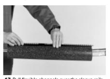
17 Pull flexible channels over the sleeve rails until they butt on top of the underclip. Centre the sleeve over the joint such that the sleeve length matches the blue lines on the aluminium foils.
