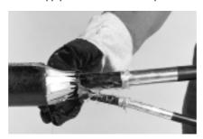
**8** Remove the PVC tape on the crowns of liner.
