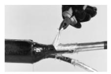
**7** Remove the aluminium flap of sleeve with a pair of pliers; if necessary reheat.
