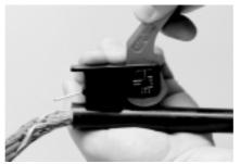
2 In order to install the shield continuity, use tool to cut the cable jacket (over a length of 20 mm and a width of 10 mm).
