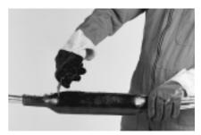
**3** Heat the sleeve circumference of the splice body and cut as shown.
