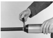
**8** Tape the crowns, starting from the liner body (10 mm) down to the cable with a 50% overlap (use heat resistant tape).
