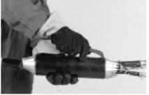
**9** Do the same at the other side. Longitudinally cut the sleeve and liner and remove both.
