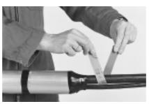
**11** Abrade the cables circumferentially over the same length as before.
