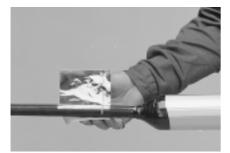
**13** Apply the aluminium foil to the cables, positioning the blue line at the mark of the bond length and smooth the aluminium foil.
