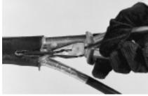
**4** Heat the clip area and remove the clip with a pair of pliers.
