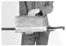
**7** Before installation of the liner, preshape the liner cylindrically by rolling. Wrap the liner tightly around the splice bundle and secure with tape.
