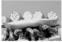
**5** Take the dessicant out of the aluminium bag(s) and place within the joint.
