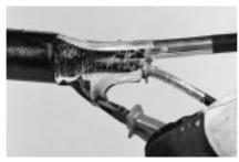
**5** Remove the sleeve end with a suitable tool by pulling the sleeve gently off the cables. Apply more heat if necessary.
