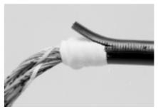
**3** Put cotton or PVC tape underneath the cable jacket strip. (see picture) Make the splice according to normal practice.
