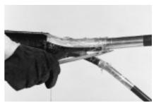
**6** While the adhesive is hot, separate the cables with appropriate tool to facilitate clip insertion when reclosing.
