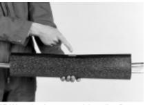
**15** Wrap the sleeve around the splice. Press the underclip (if applicable) over the rail at the centre of the sleeve.
