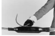
**2** Cut off the channel starting from the cable end up to the centre of the splice, to avoid cable cutting.
