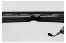
20 Start heating in the centre of the sleeve 180 degrees from the channel area. Continuously heating circumferentially (heating equally on both sides) until arrival at the channel area. The recovery in the channel area should take place towards the end of the installation. Continue heating until the thermoindicating paint has changed colour from green to black.
