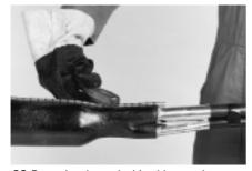
**22** Press the channel with a blunt tool to give the channel the shape of the liner transition.
