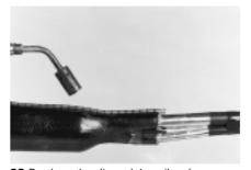
23 Postheat the clip and the rail and channel area at the cable ends.
