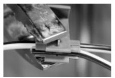
**6** For joints with three or more cables, install continuity wire on shield continuity wire assembly using crimp connector.
