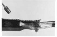
**21** When temperature sensitive paint has completely changed to black, gradually and progressively move towards the end of the sleeve.
